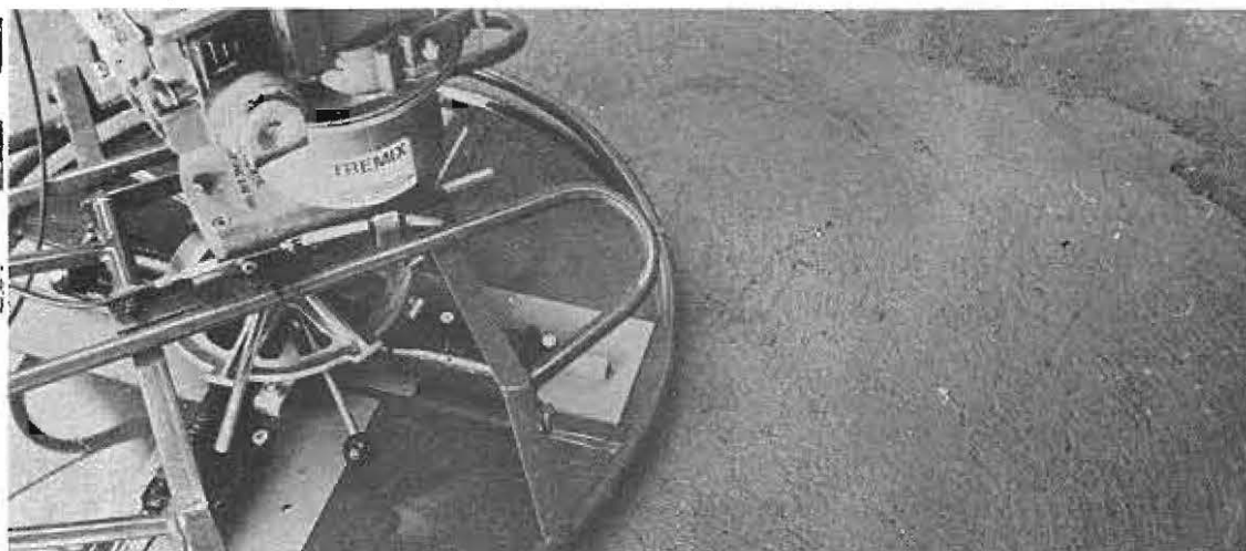
Fig. 12 CLASS U2 FLOATED (POWER). NOTE: THE FINISH SHOWN IS PRODUCED BY A DETACHABLE STEEL REVOLVING DISC MOUNTED BELOW THE TROWEL BLADES
